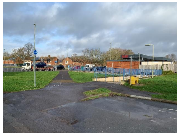
Photograph 4: Petersfield Road Subway
