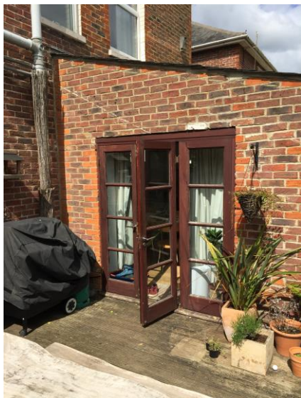
Existing doors from dining room
