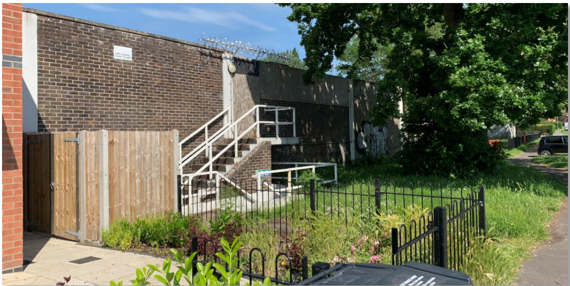
Fig 05: Existing brickwork and escape staircase on the east of the car park
