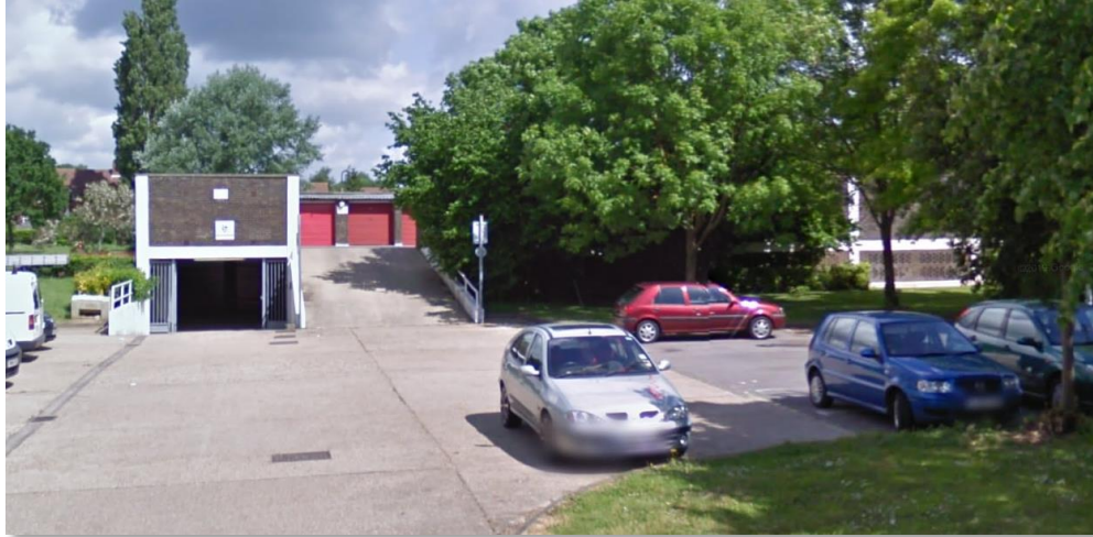
Fig 04: Existing building on site [source: google maps]
