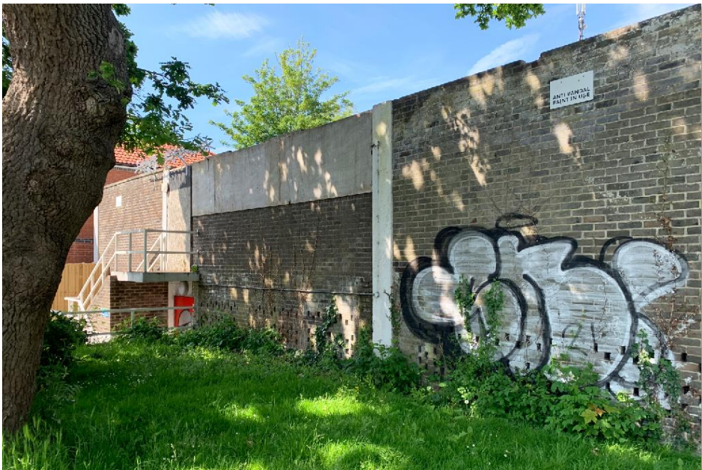
Fig 08: Existing brickwork and escape staircase on the east of the car park
