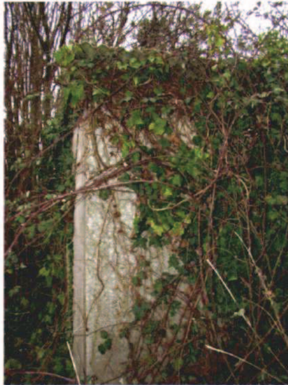
Figure 2: concrete-built single-storey storage outbuilding (B2)
