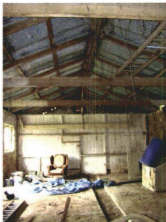
Figure 3: Stable block structure open to the rafters and unlined (B1)
