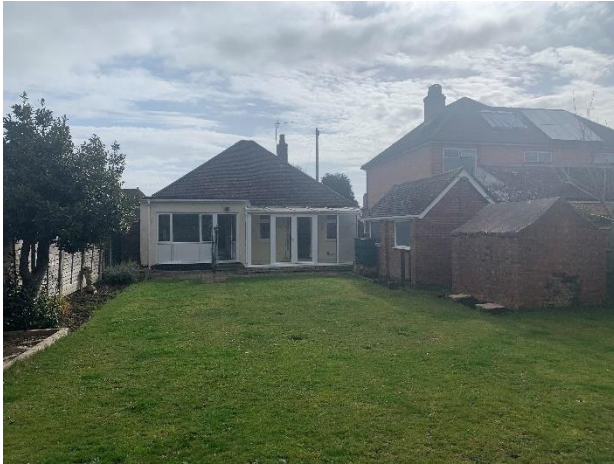
Figure 3: Rear Elevation of dwelling
