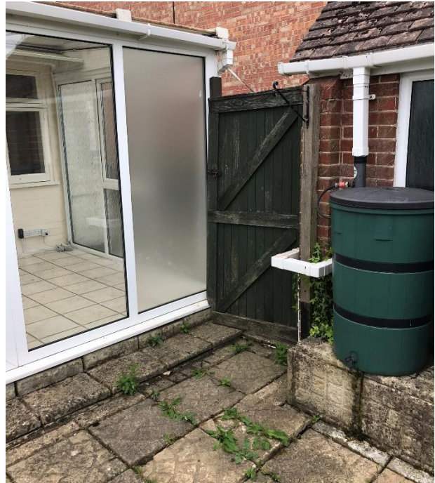
Current side access between lean-to and garage.
