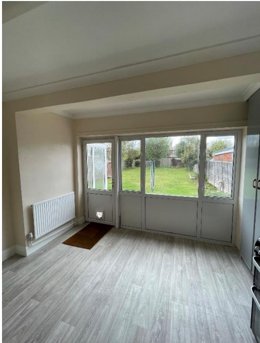
Existing rear extension.
