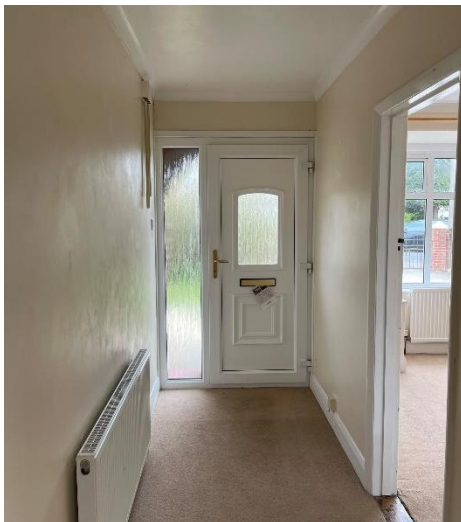
Existing main entrance.
