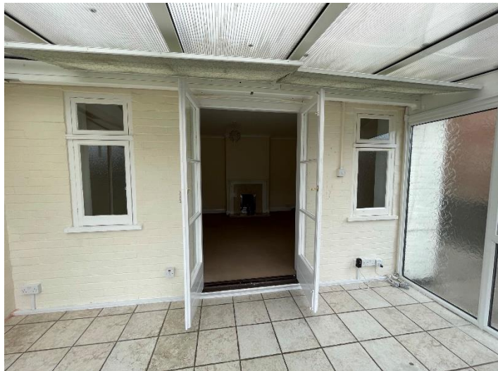
Doors between current lean-to and main dwelling.
