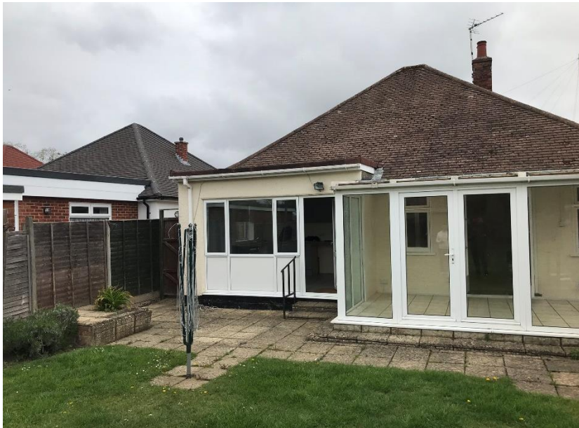
Existing extension and glazed lean-to that are proposed for removal.
