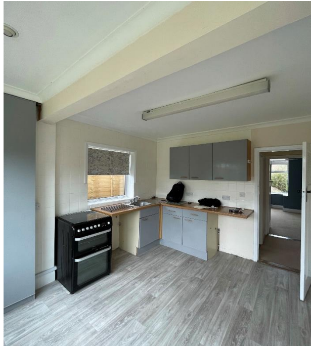
Existing kitchen to be renovated and extended.
