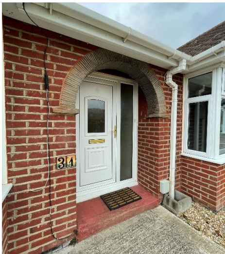
Existing main entrance.
