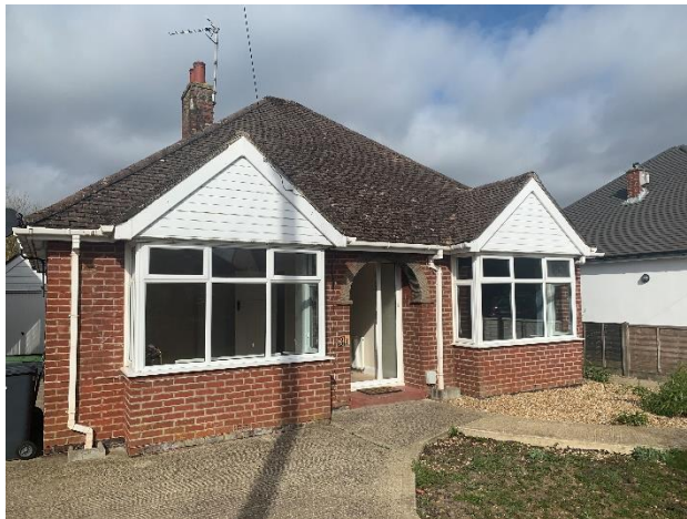
Figure 5: Front Elevation of dwelling
