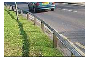
TYPICAL KNEE RAIL FENCING TO PAVEMENT
