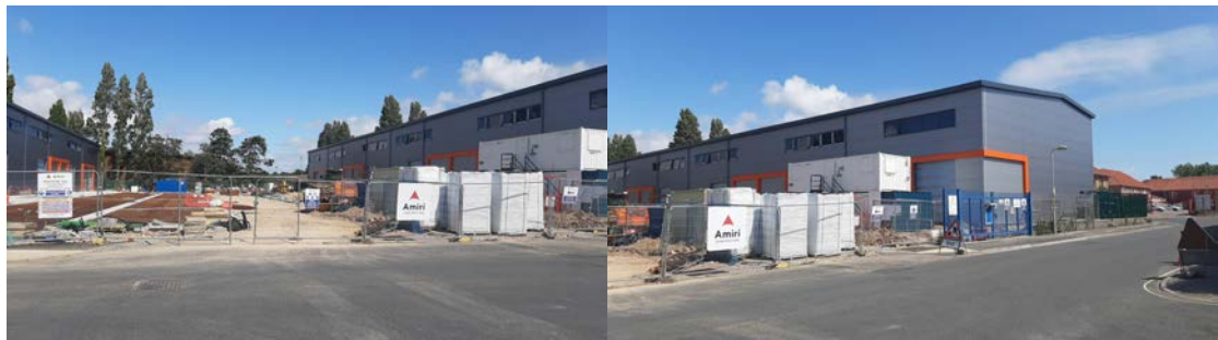
Stanbridge Road new site entrance under construction (August 2021)
