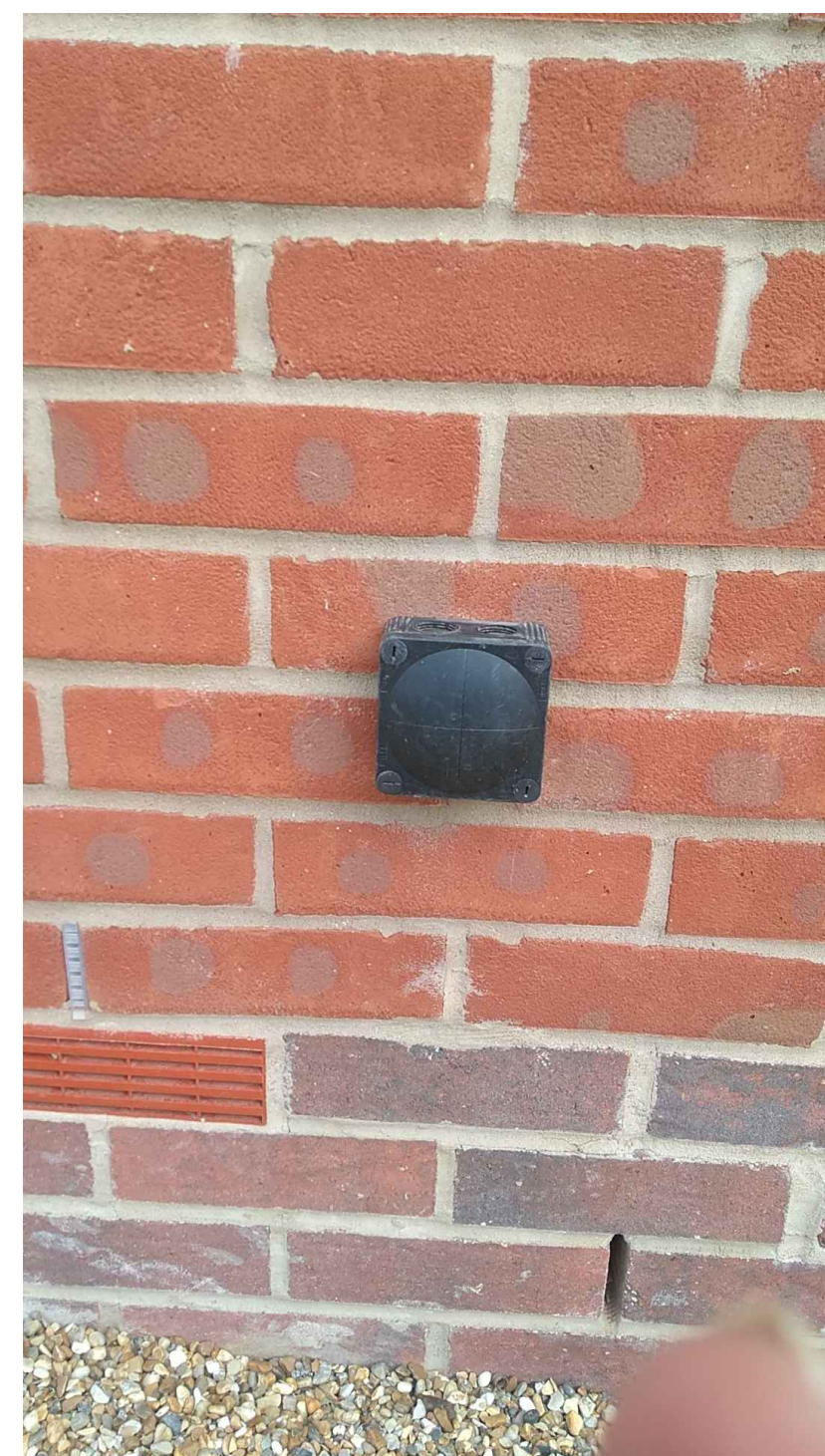
WISKA Polypropylene Junction box (Photo as installed)
