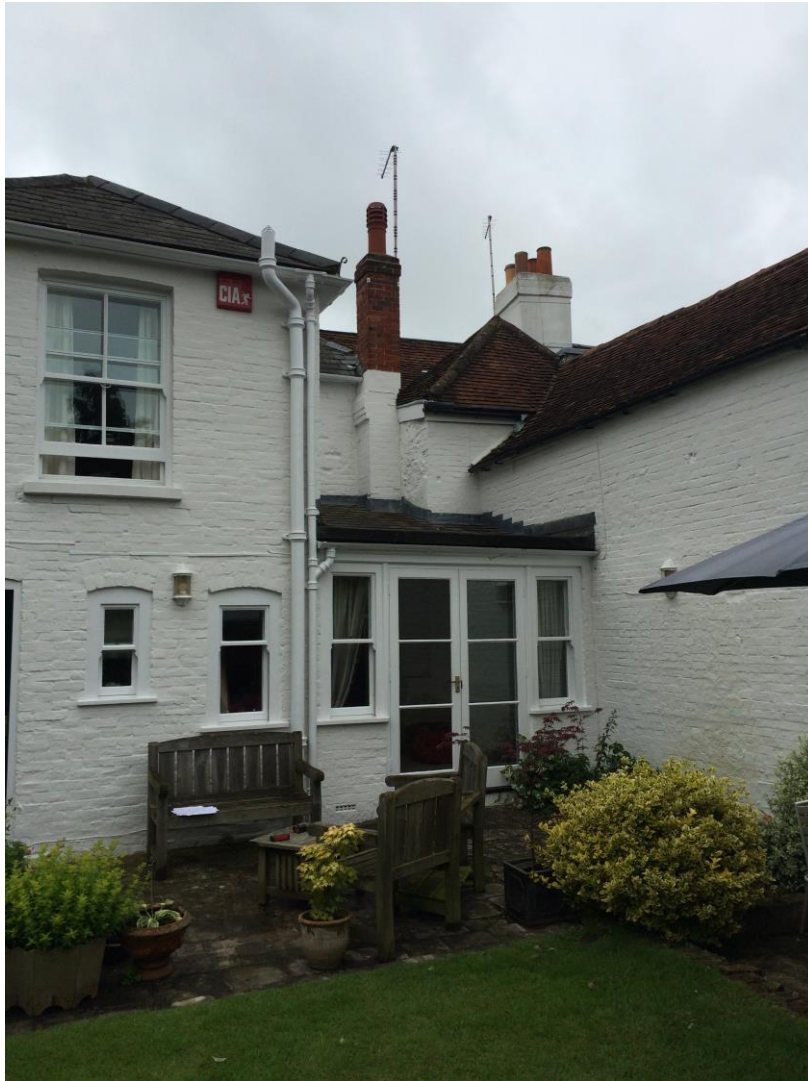
View from the garden showing doors and roof to be replaced in context
