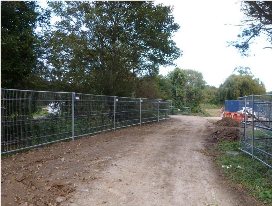
Illustrating the pinch point access into the site from the Works Compound into the Main Development Site.
