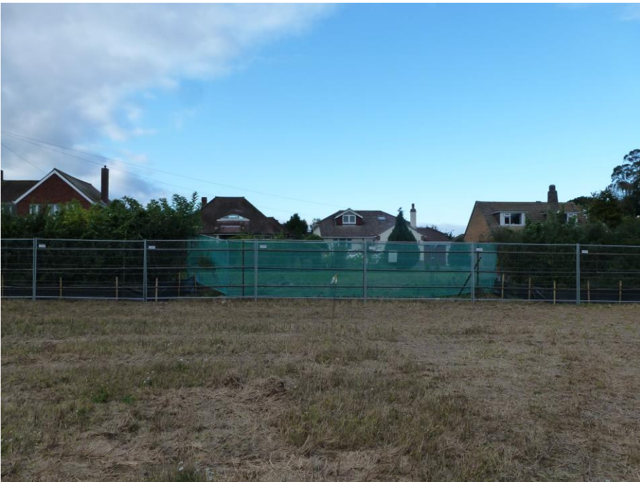
Illustrating the fencing off for the Hedge 1 frontage but allowing for the new access point to be formed (green netting).
