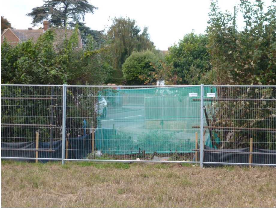
Illustrating the fencing off for the Hedge 1 frontage but allowing for the new pedestrian access point to be formed (green netting).
