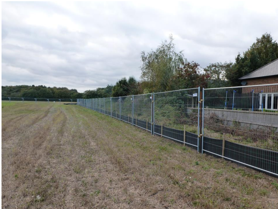
Illustrating the fencing off for the western boundary abutting existing residential property.
