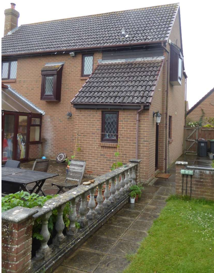
3.Rear (east) and side (north)
