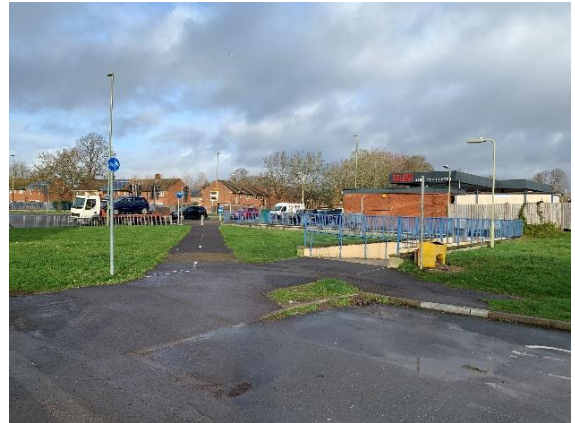
Photograph 2: Petersfield Road Subway
