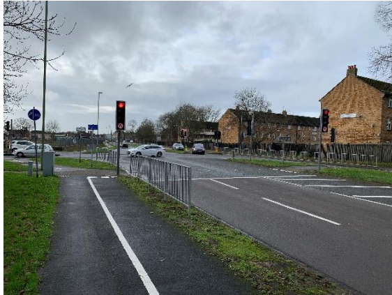
Photograph 1: Petersfield Road Pedestrian Crossing
