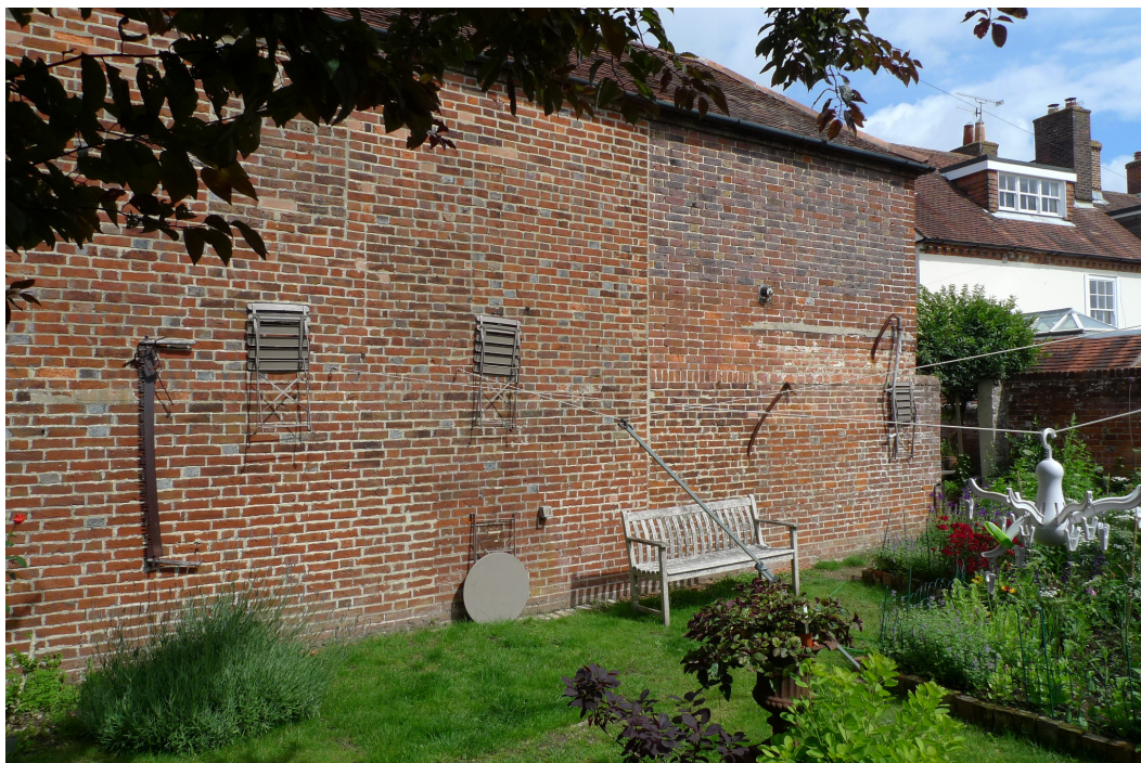
Photo of the South elevation of the annexe (previously a grain store). Note it has undergone several alterations as seen in the mis-match of brickwork and infilled openings.
