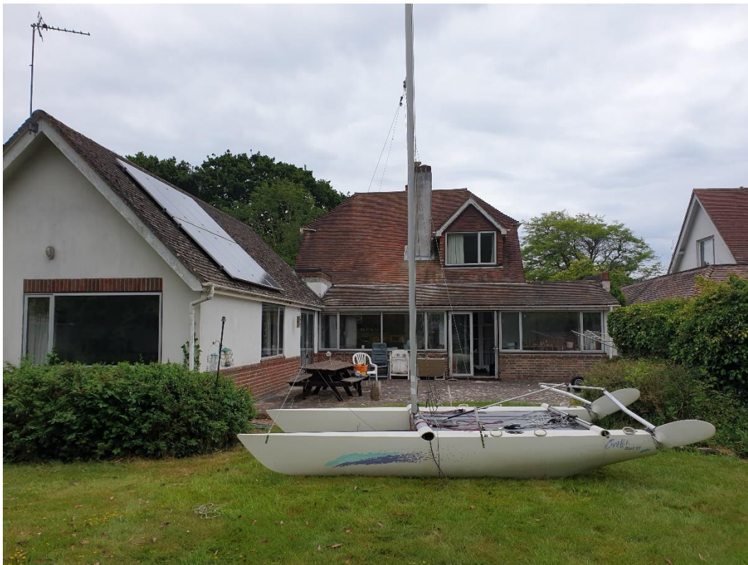
48 Sinah Lane – Rear view
