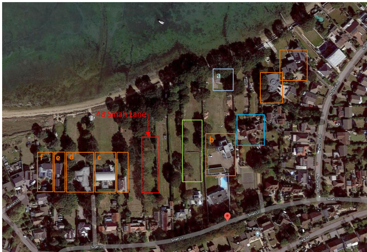
Fig. 1 – Dwellings constructed midway on plots behind dwellings fronting Sinah Lane, Dwelling set midway on the plot with no dwelling fronting Sinah Lane, permission for separate dwelling midway on the plot (No. 42), outbuilding in garden.
