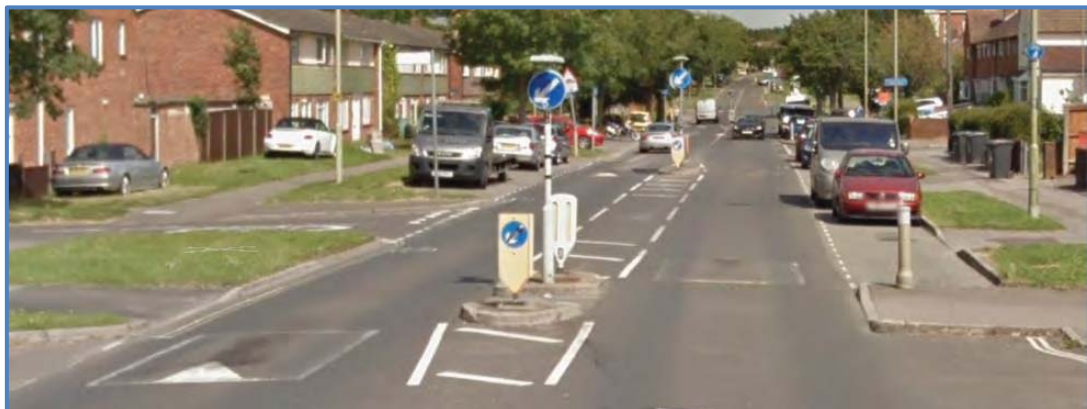
Photo 2.3 – Crossing with dropped kerbs on Dunsbury Way, close to Bishopstoke Road.
