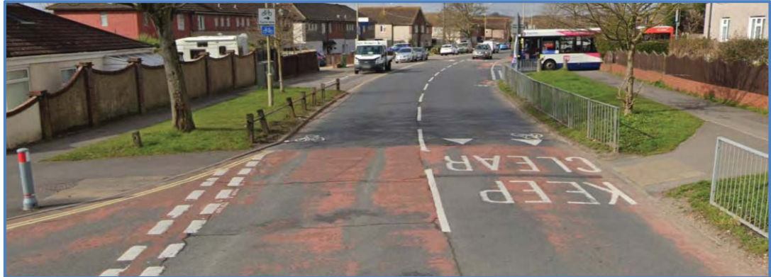
Photo 2.2 – Tactile paved crossing on Middle Park Way, east of Swanmore Road junction.
