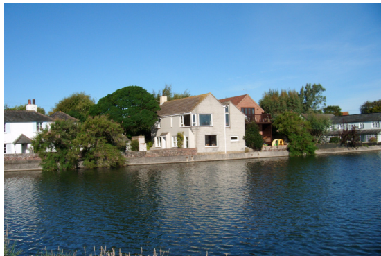
Photo showing the view of the application property from the Mill Pond
