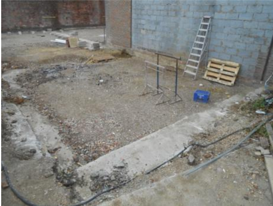
Backfilled with crushed concrete
