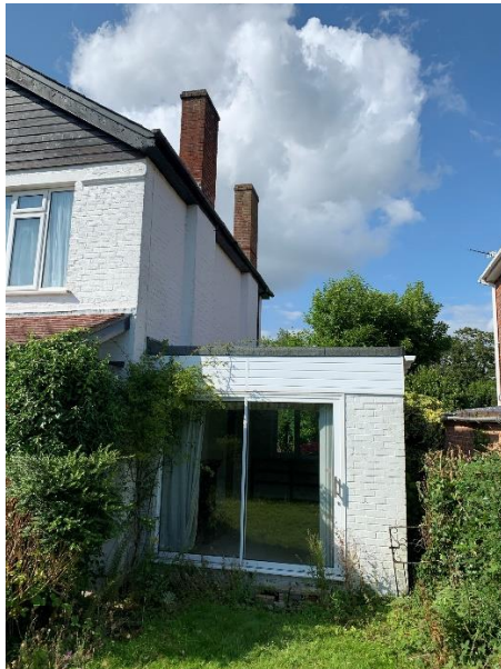
Figure 5: Existing eastern side extension
