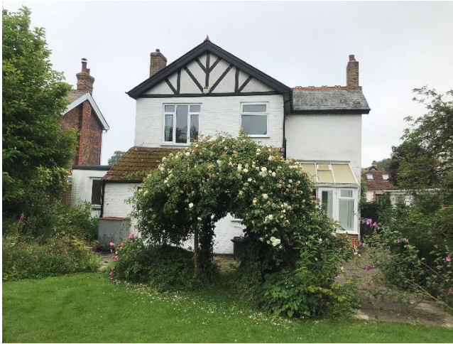
Figure 3: Rear Elevation of dwelling
