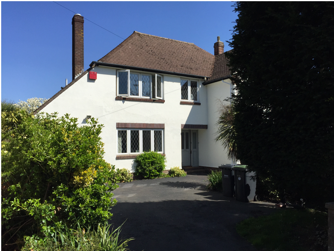
Figure 1: View of property
