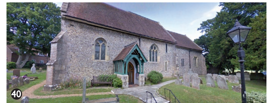
40 Church of St Thomas, Bidbury Lane, Bedhampton (Grade II listed, dates from 12th century with various alterations made later)
