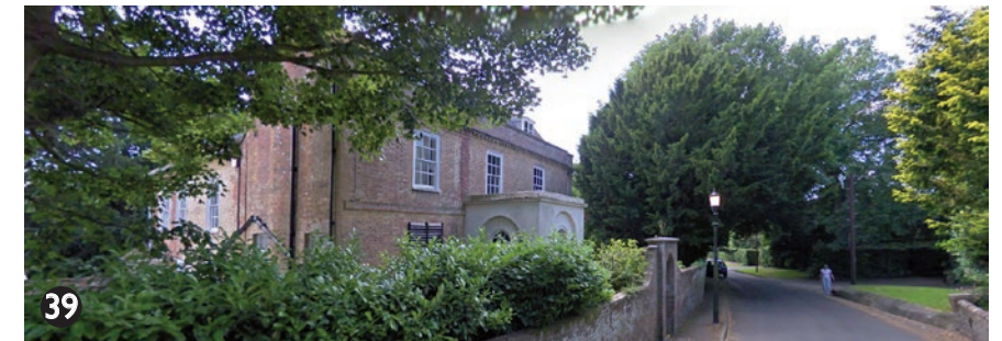
39 Old Rectory, Bidbury Lane, Bedhampton (Grade II listed, dates from late 18th century)
