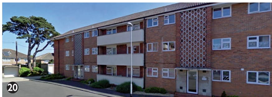
20 Three-storey apartment block on East Park Lodge, Farlington (dating from circa 1970)
