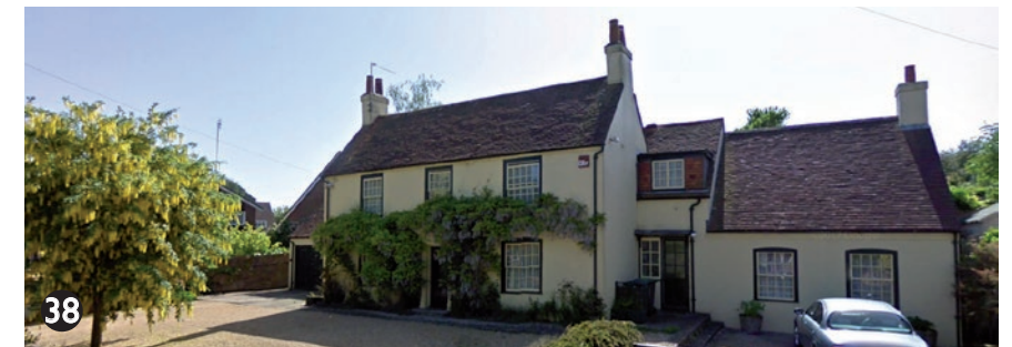
38 Grade II listed house known as 'Spring Lawn' on Brookside Road, Bedhampton. Dates from early 19th century.
