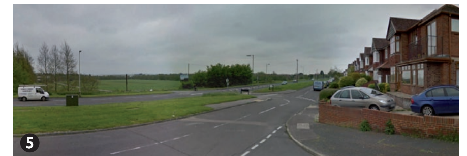
View west along Auriol Drive and Havant Road from the junction between Auriol Drive and Fortunes Way
