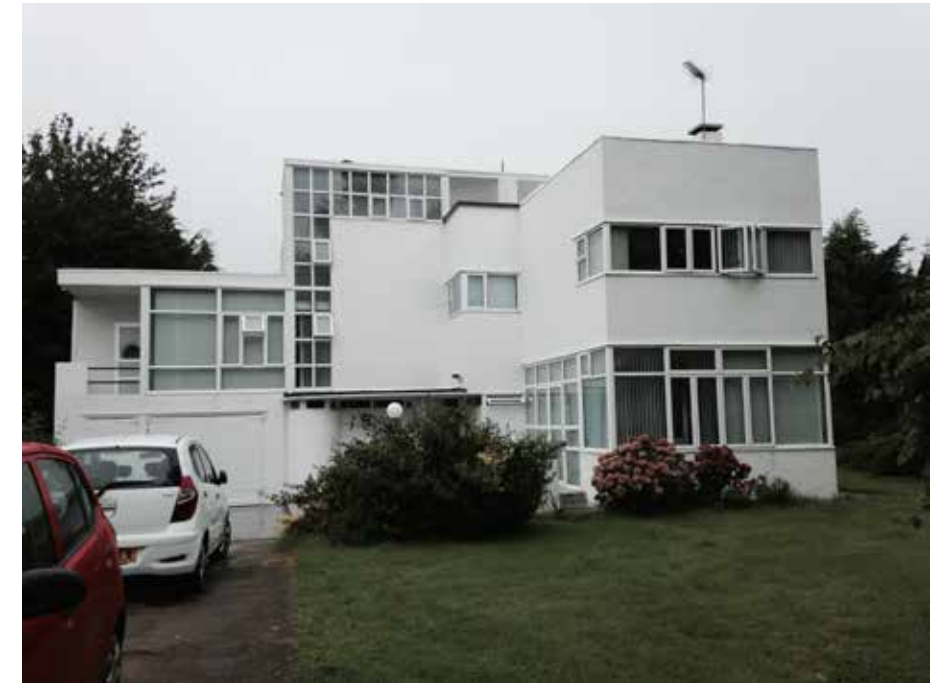
Front elevation and (south facing) garden of Saltings, which the ground floor living space face onto
