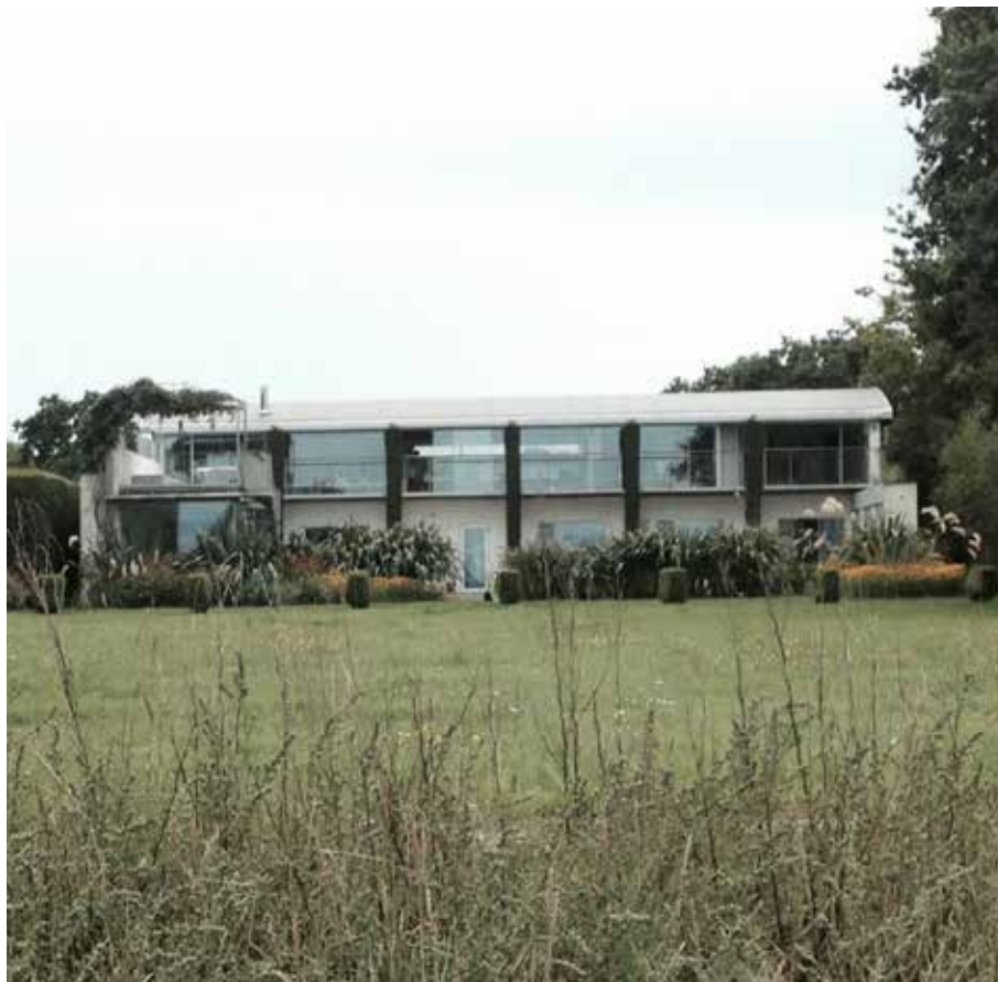
4. House to the rear of 52 Sinah Lane
