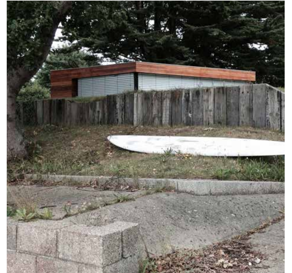
3. Outbuilding to 40 Sinah Lane
