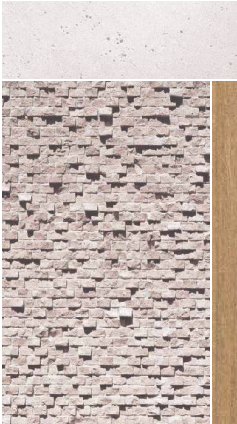
Textured brickwork walls
