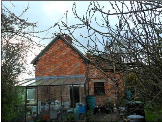
Photo 9 – Holly Bank Farm House
