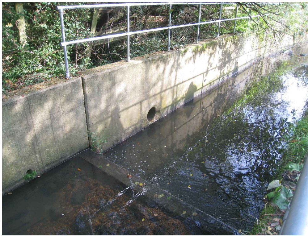
PHOTO 1 LOCATION OF EXISTING OUTFALL ON THE LEFT BANK
