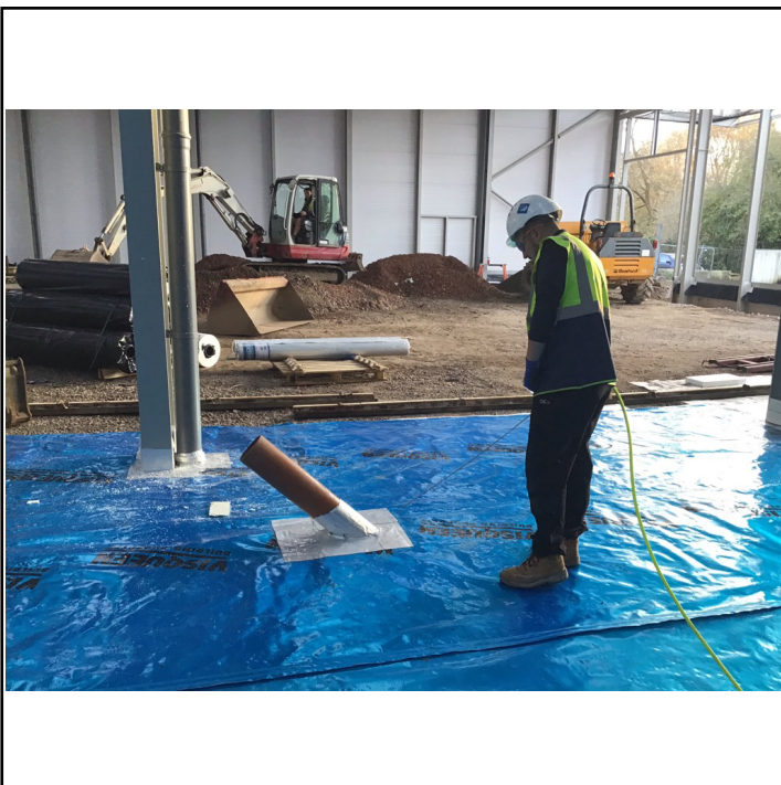
Air lance integrity test carried out to pipe detail.
