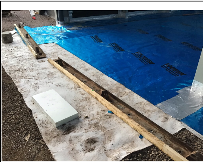
Protective fleece applied under the membrane.
