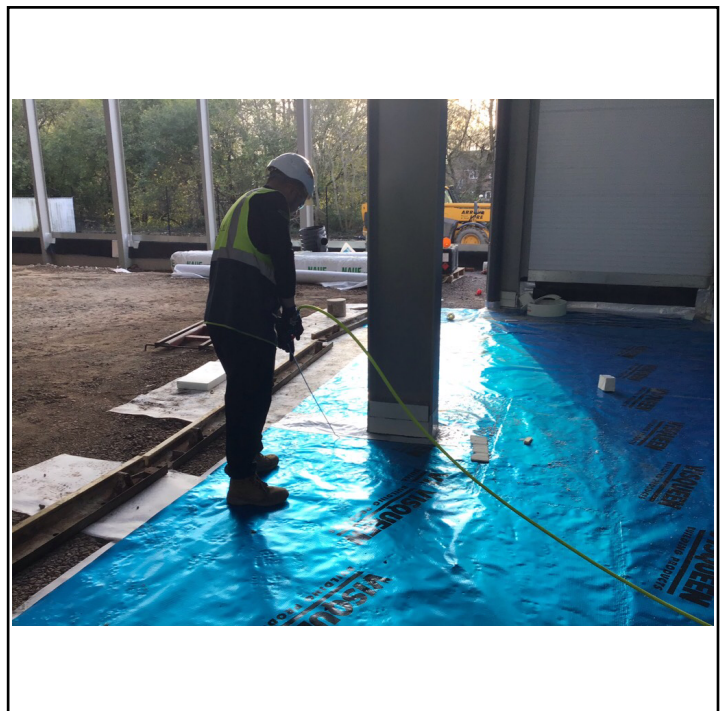
Air testing to steel stanchion.
