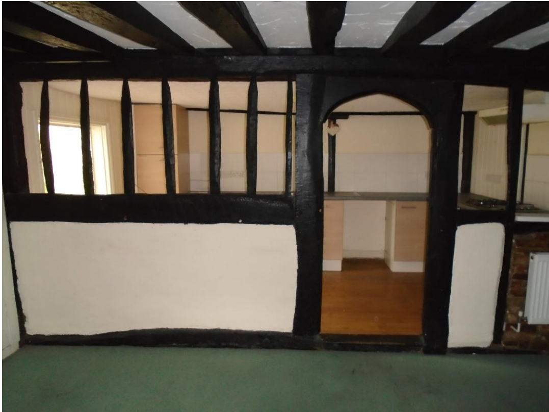
Figure 3. Timber framing and studs in Unit 2 would be retained.
