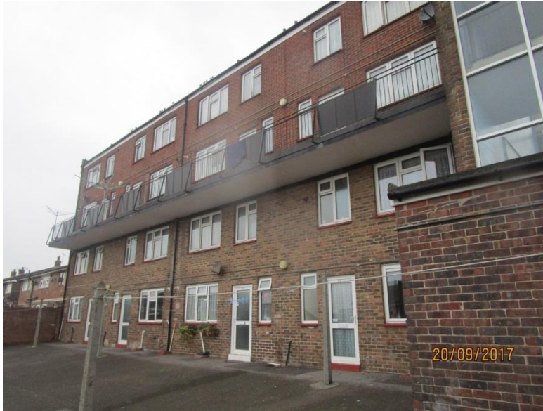
Photo 3 - Rear elevation showing balcony walkway
