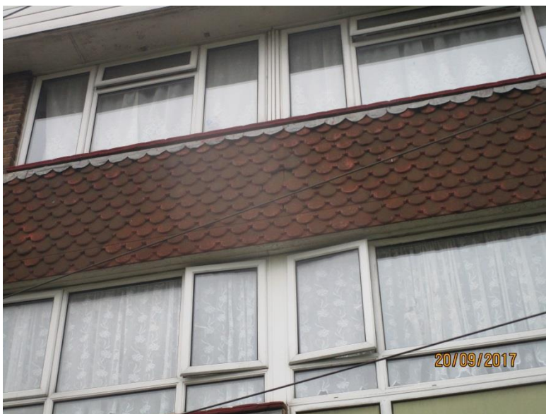
Photo 5 - Tile hanging to front elevation
