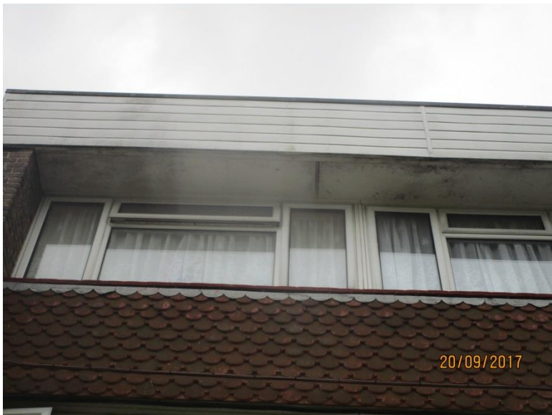
Photo 4 - Existing Fascia Board and Soffit
