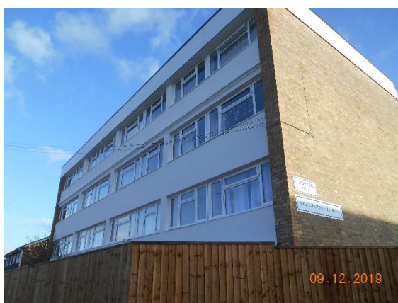
Similar Completed Pilot Block (Prospect Lane)
