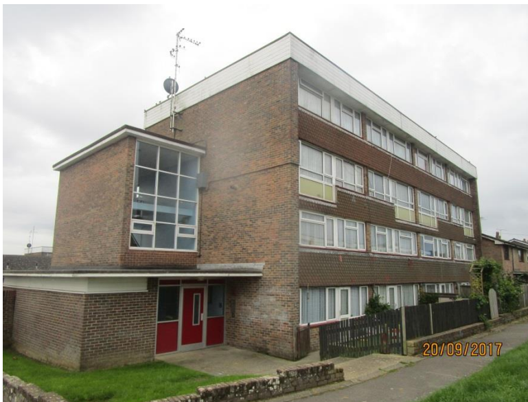
Photo 2 - Front Elevation showing boundary fencing
