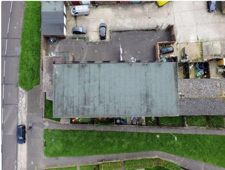
Photo 1 - Aerial view of the block
