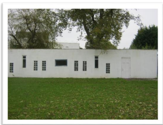
Flat roofed structure to be demolished. Unsuitable to bats owing to the open void roof.
