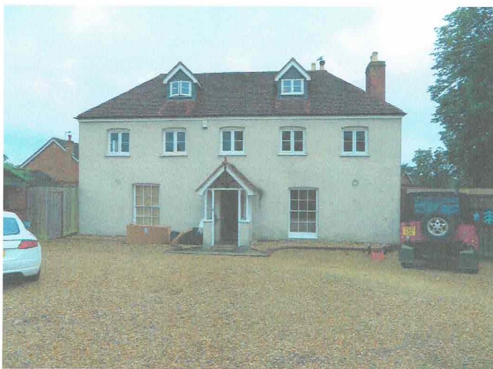
Front elevation of 'The dairy House'
