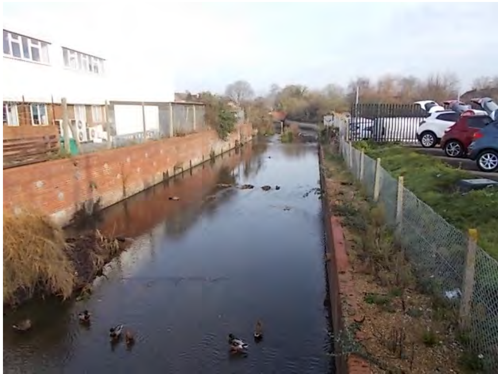
View from West street bridge towards railway bridge ( site beside/behind car lot to RHS)
