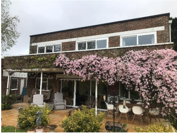
Figure 4: Rear of existing property
