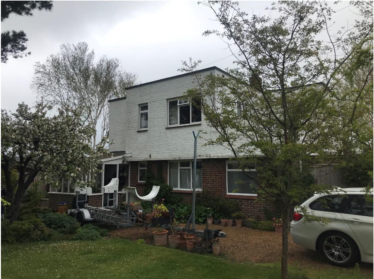
Figure 1: View of existing property entrance
