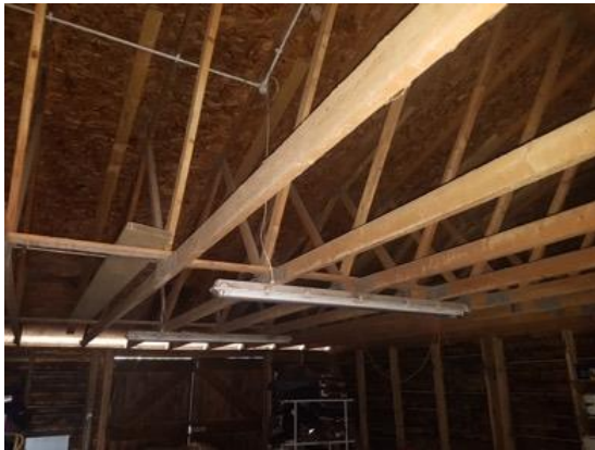
Photo 10: Internal view of roof structure showing exposed timber beams. B2.
