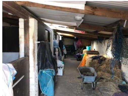
Photo 21: Internal view of B5.
