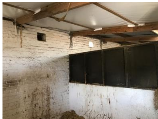
Photo 23: Internal view of stable block, B5.
