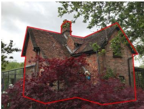
Photo 31: Red line highlights B8. North-facing elevation.
