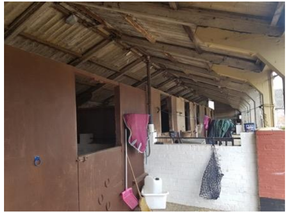
Photo 17: Internal view of B4.
