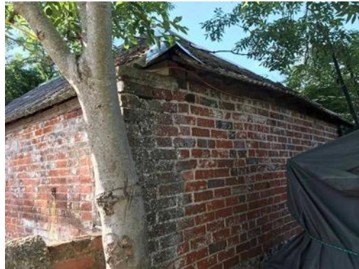
Photo 13: Rear north-facing elevation of B3.
