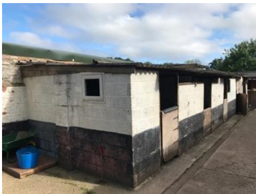
Photo 22: West facing element comprising of stable blocks. B5.
