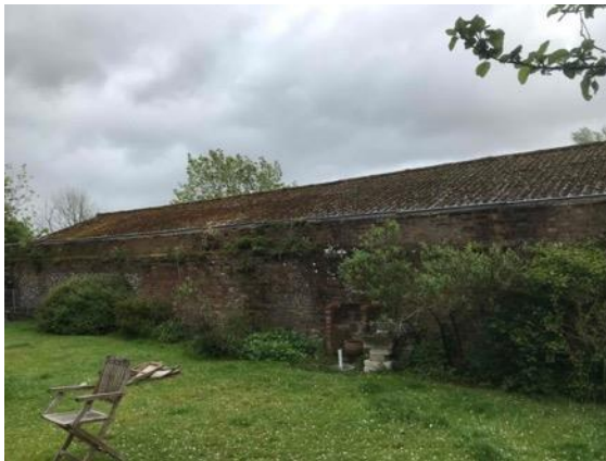
Photo 18: Rear north-west facing elevation. B4.
