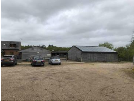
Photo 1: View of timber stable block and compacted gravel parking area.
