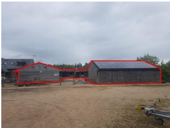
Photo 8: Red line highlights survey building B2.
