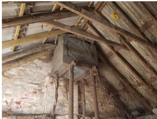
Photo 15: Internal view of roof structure. B3.
