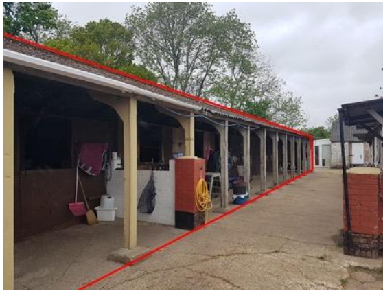
Photo 16: Red line highlights survey building B4.
