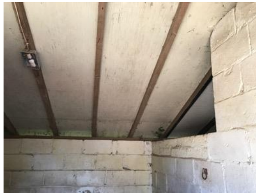
Photo 25: Internal view roof structure. B6.
