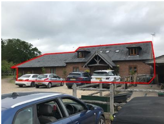
Photo 1: Red line highlights survey building B1. Front south-facing view.
