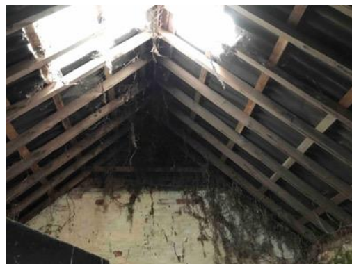
Photo 30: Internal view of roof structure. Main element. B7.
