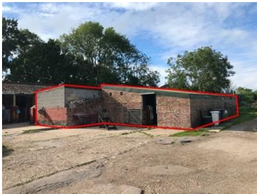
Photo 20: Red line highlights survey building B5, showing south-facing elevation.
