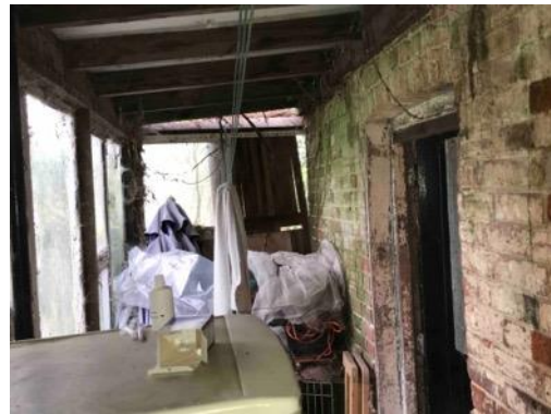
Photo 28: Internal view of mono-pitched element. B7.
