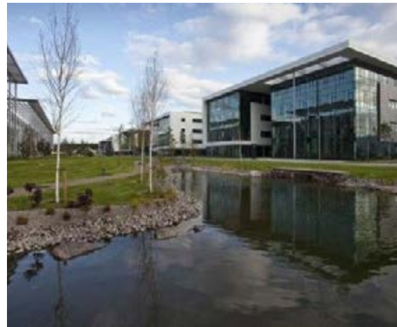
Swales and attenuation form drainage and maintain the natural habitats of local wildlife
