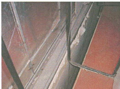
Single skin plasterboard partitioning
