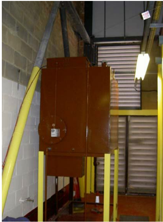
Photograph 5: Back-up generator diesel storage tank
