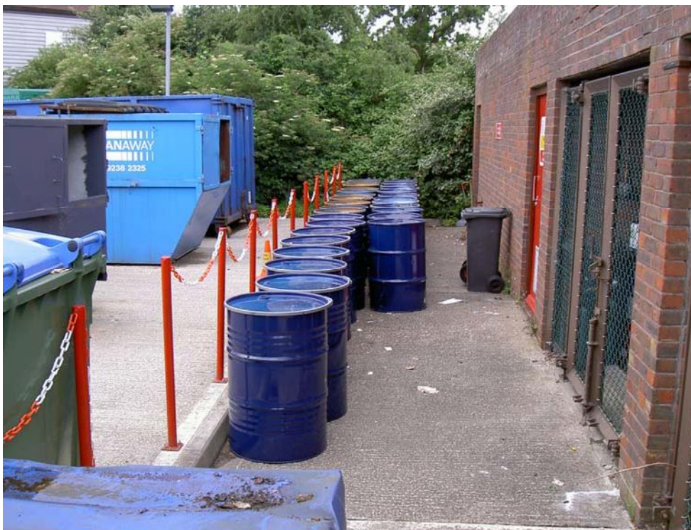
Photograph 12: Drums containing contaminated rags and PPE
