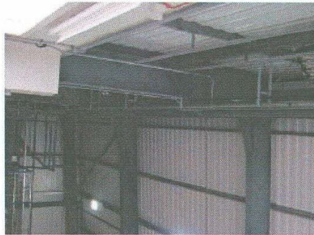
Steel girders and metal sheet roof
