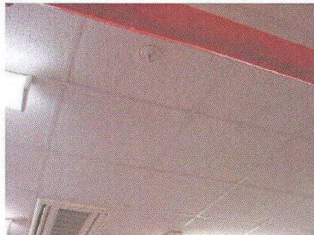
Compressed board tiles in 1st floor office
