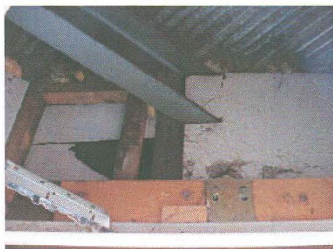
Supalux board in void of security block
