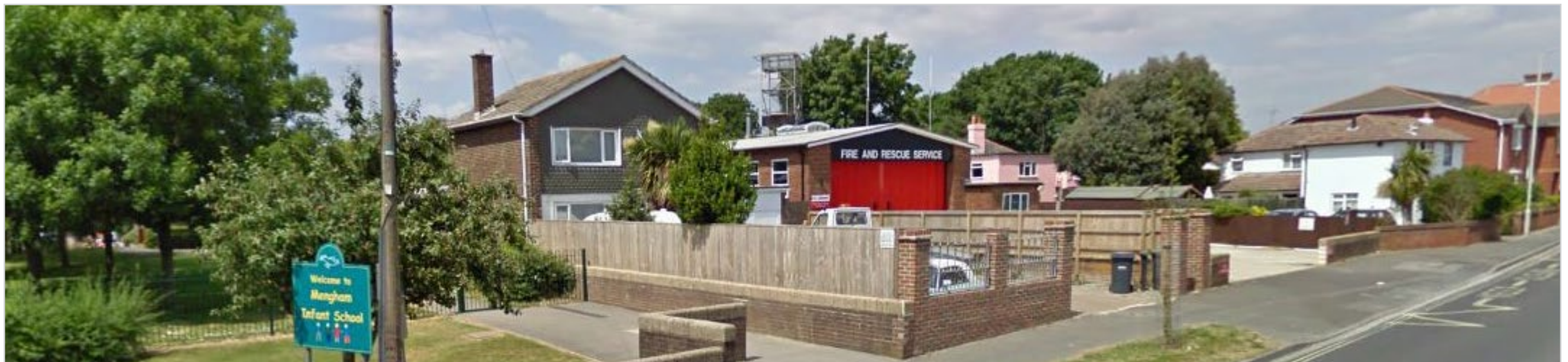
view along west side of Elm Grove - open character
