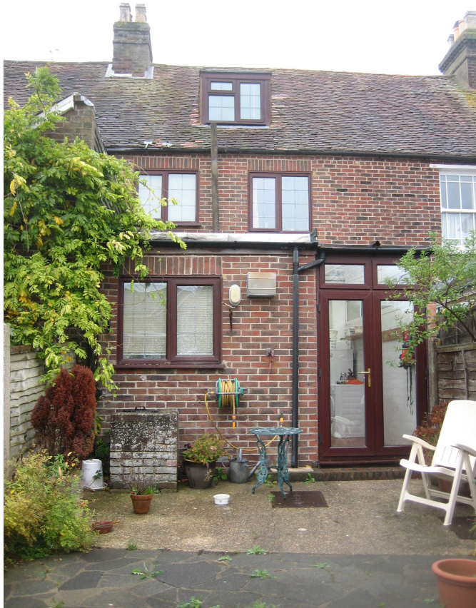
Fig 2 – View of existing single storey rear extension .
