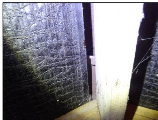
Figure 9 – exposed roof and ridge tiles between the bitumen lining and the ridge beam of the roof void
