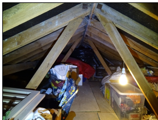
Figure 7 – internal view of the roof void, looking north
