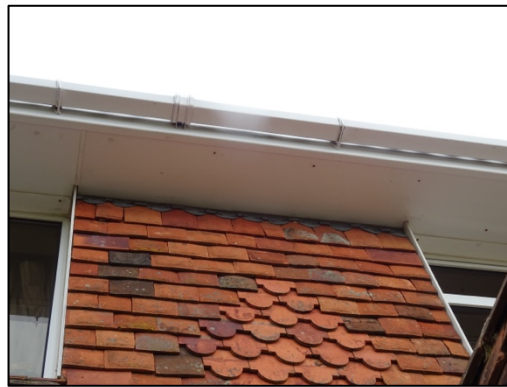
Figure 5 – plastic underboards enclosing the eaves on the western elevation of the house
