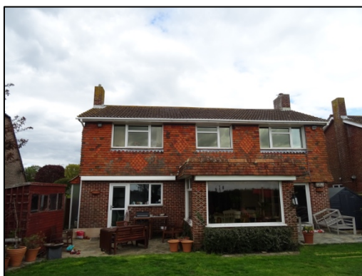
Figure 4 – western elevation of the house with the single storey extension
