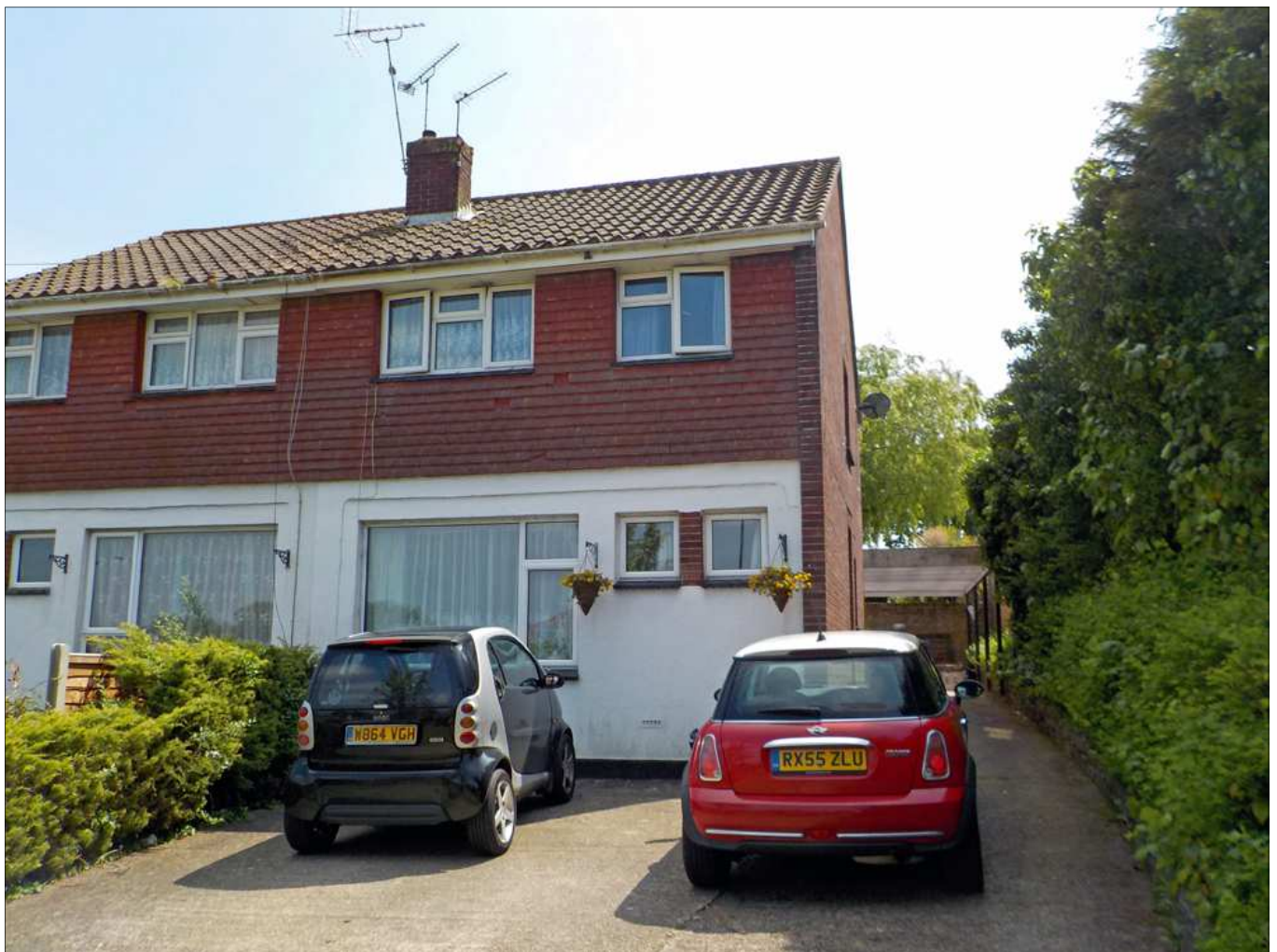
Front of No. 52 London Road
