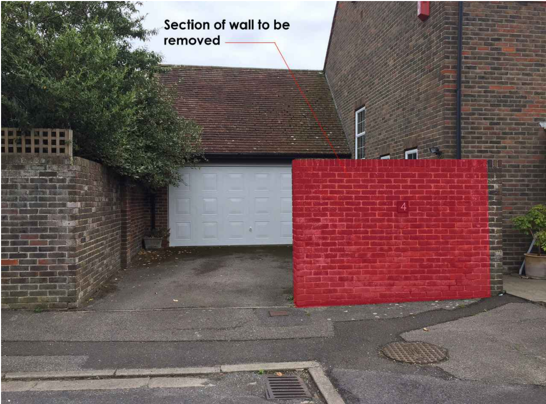
Photo of Existing Wall
