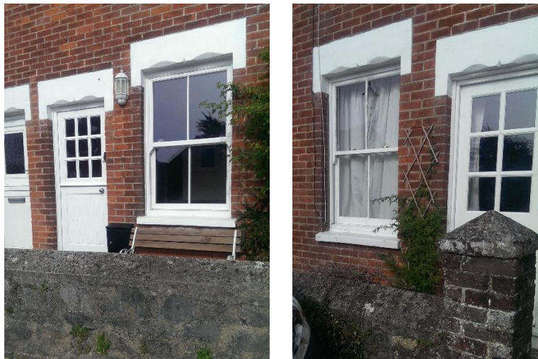
Windows on surrounding buildings.
