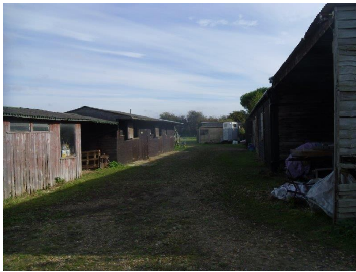
View looking east to existing stables, barns and yard
