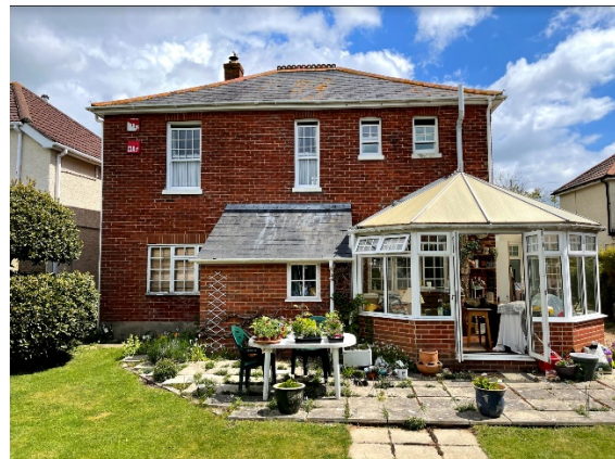
Figure 02: Rear Elevation showing extension and conservatory
