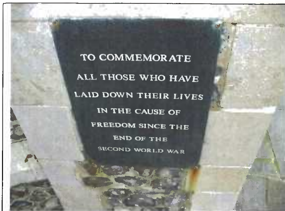
Generic plaque commemorating Post 1945 lives lost but also the rusting caused by incorrect fixings at the base of the plaque
