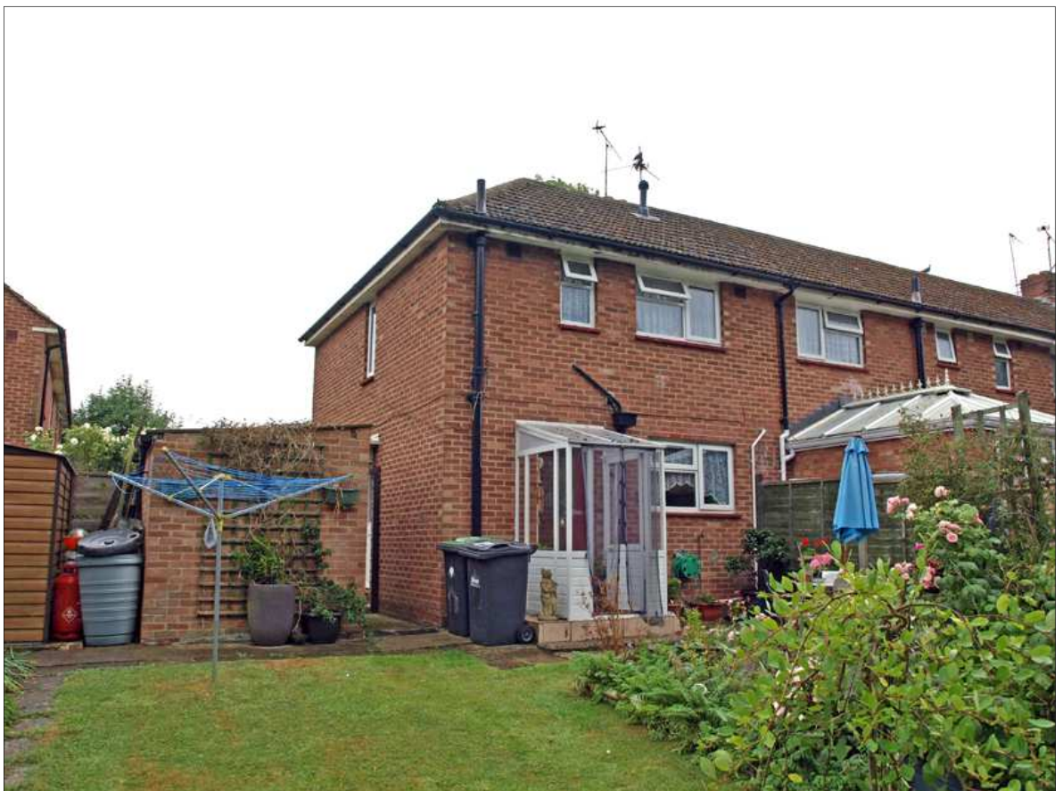
Rear view of No. 23 Highlawn Way
