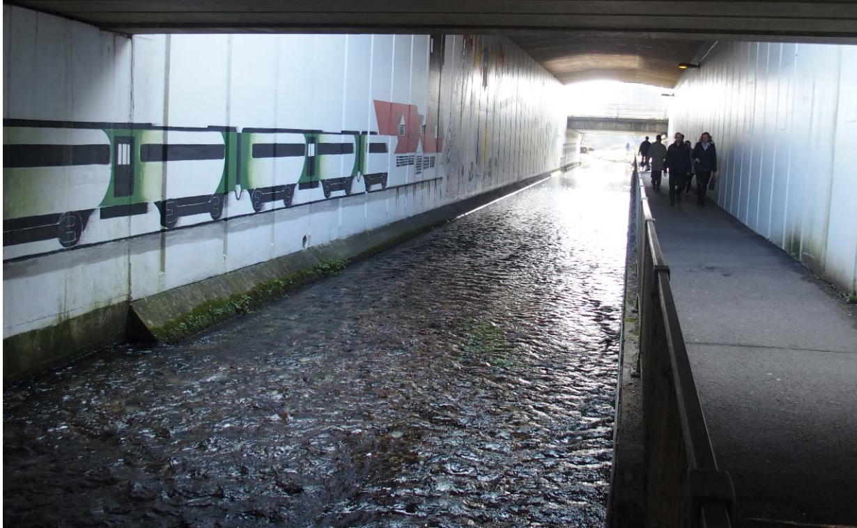
Photograph No. 09 - Canalised section of the watercourse approximately 90.0 metres downstream of the site.
