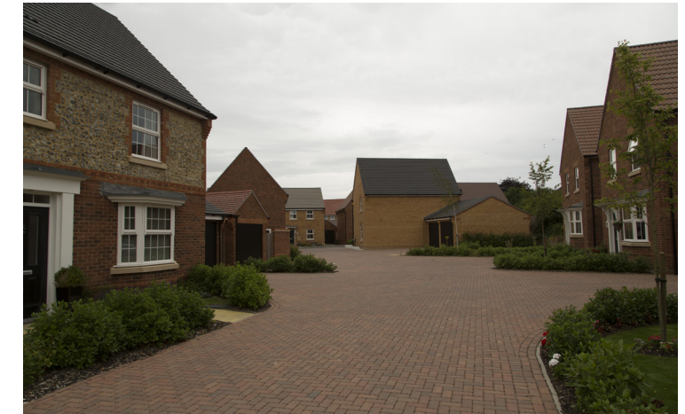
Shared surface within the David Wilson Development
