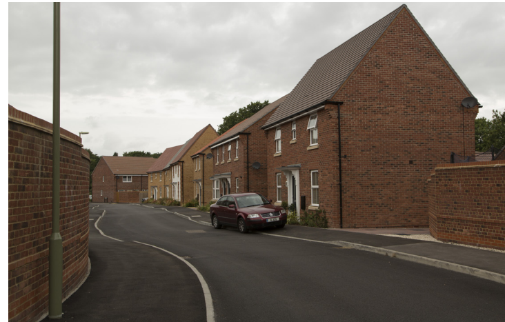
Front, side elevations and gables within the David Wilson Development
