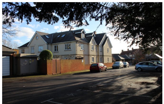
Photo 4: Apartment block located on the corner of Station Road and the private access road (un-named)
