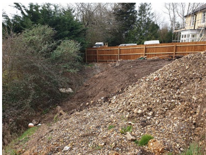
View from eastern garden looking west showing mound of spoil.
