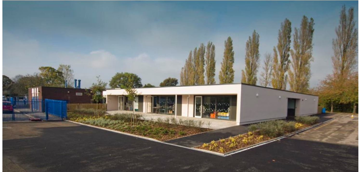
FIG 2: Existing Site Photograph.
