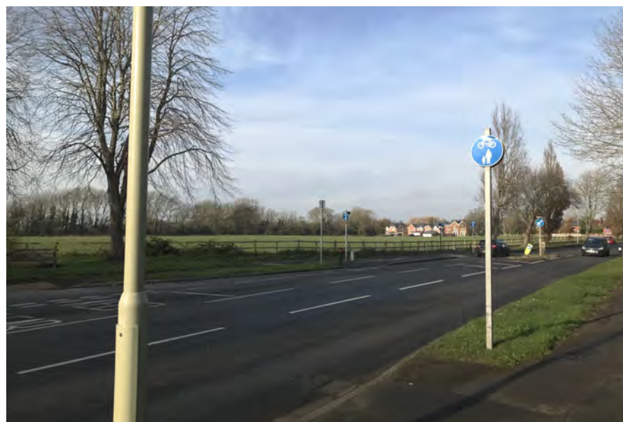
Figure 11: View across Site looking north west.
