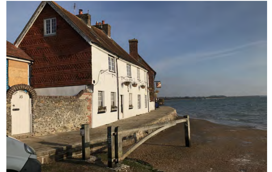
Figure 20: View of Grade II 16, 17, 18 Langstone High Street with Grade II Royal Oak Public House partly visible behind.
