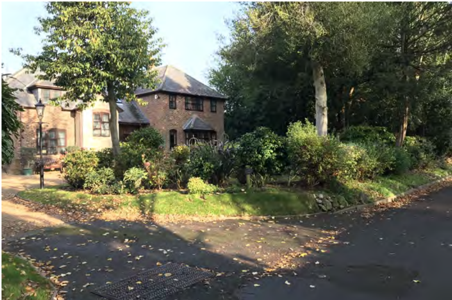
Figure 18: Example of typical residence on north side of Mill Lane, looking north east.
