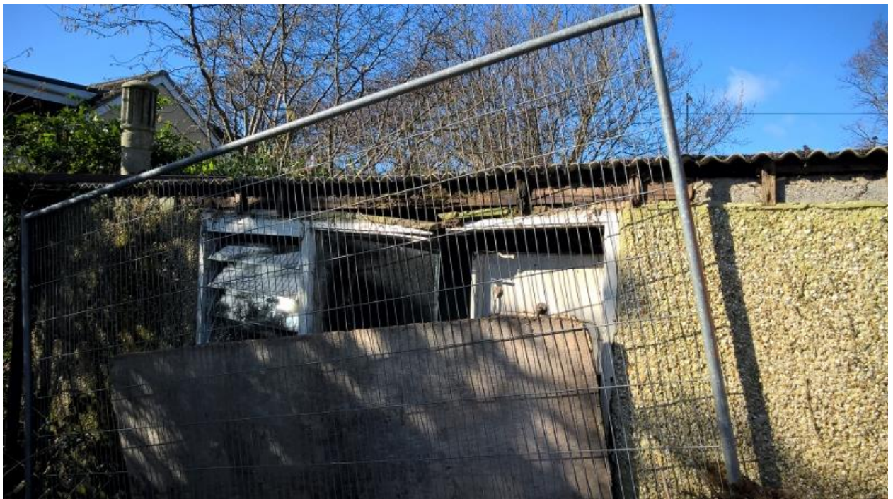
Plate 6: The rear of the garage block that is to be demolished to allow for an access road
